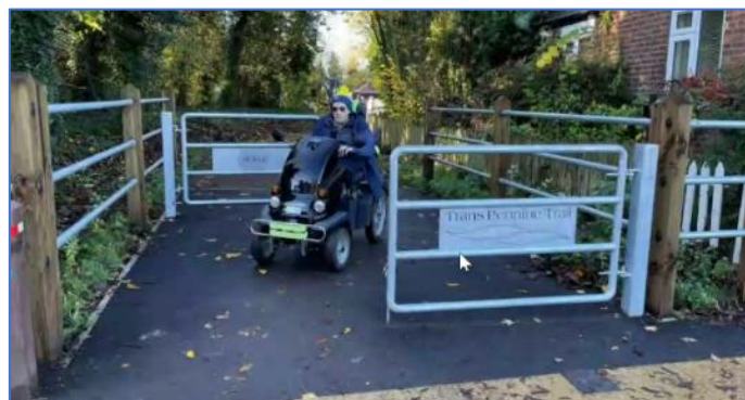
Figure 5: Chicane with 3.5m spacing on the Trans Pennine Trail
