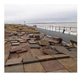
Looking at ways to protect the coastline at Crosby where the Sea wall is beginning to fail. The rubble beach also needs work as waves are eating away at the coastline causing it to move inland. There are also some homes at risk from surface water flooding and we are looking at ways to lower their risk.
